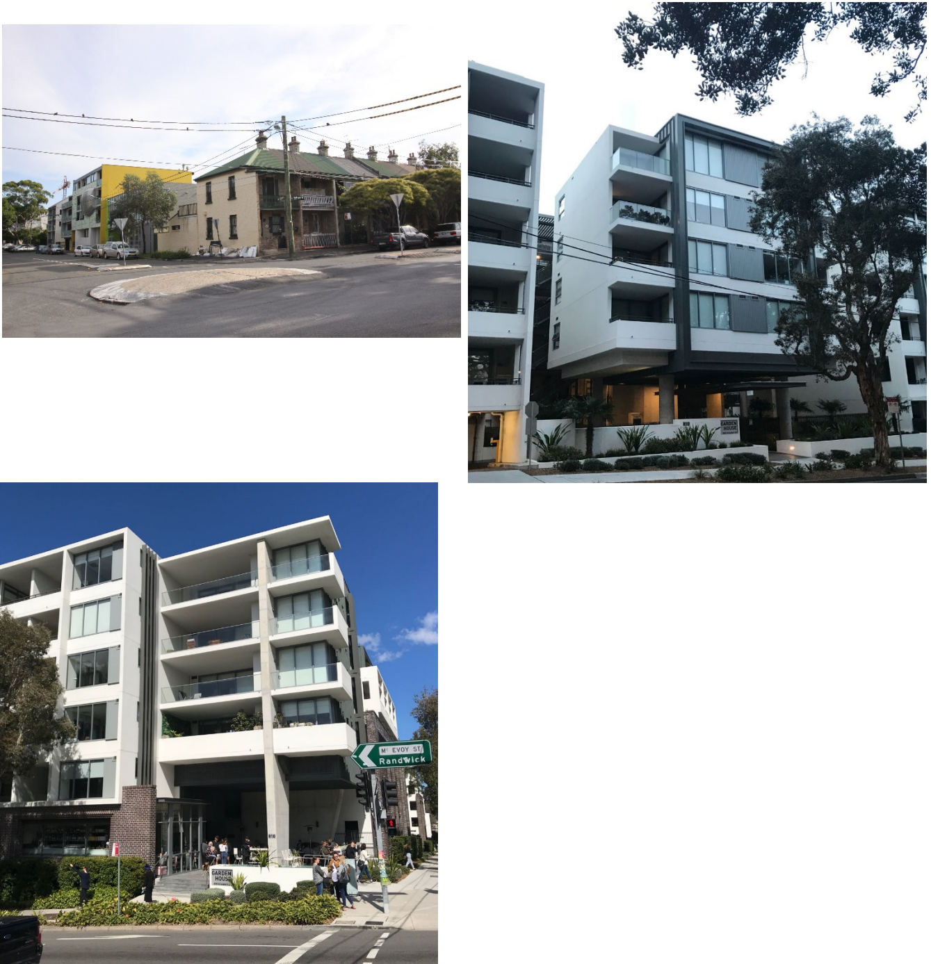
Figure 4 Built form character in the surrounding area
